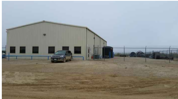
Typical O&M Building and Side Yard
