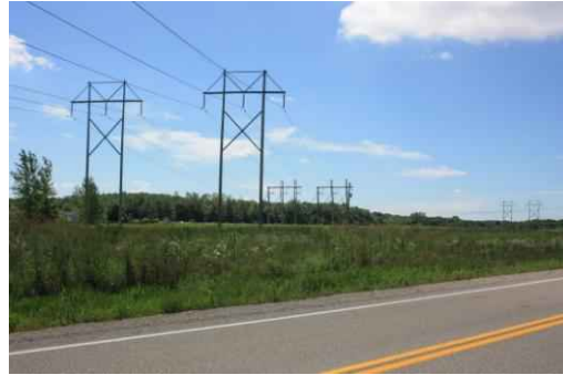
Existing Transmission Line
