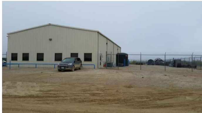
Typical O&M Building and Side Yard
