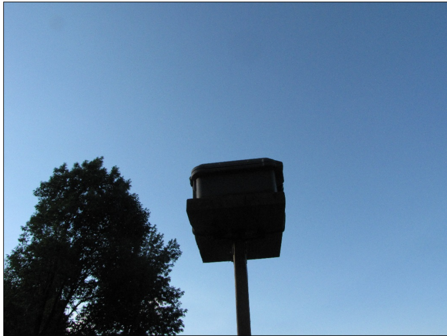
Site 6-A (Canopy; facing north)
