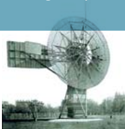
1888: Charles Brush develops first large wind generator producing 12 kW DC
