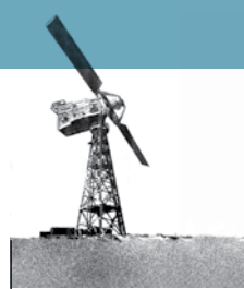
1941: Putnam's 1.25 MW turbine demonstrates need for lighter materials
