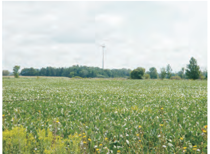
Plate 8 Wind Turbine, View Southeast from Danceland Road East of Blackbush Line
