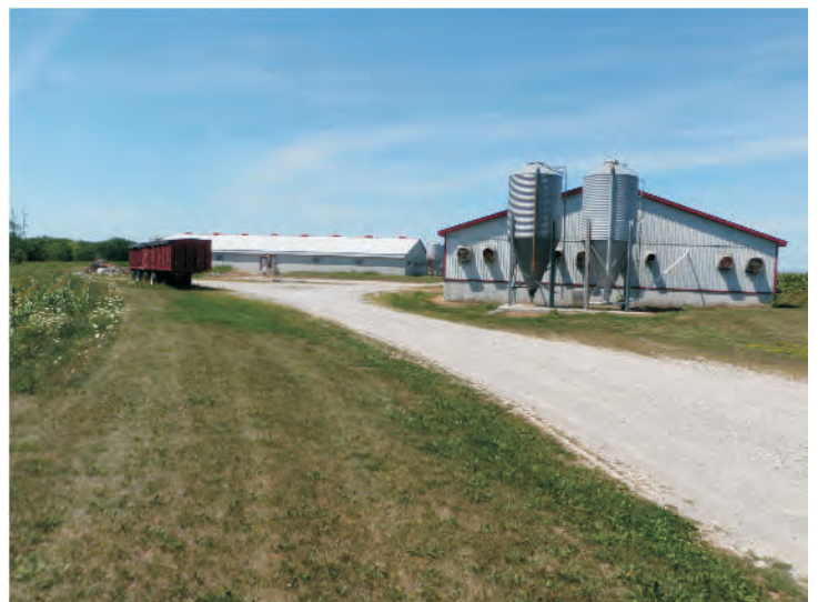
Plate 12 Proposed Access Road to Turbine 44, View Northwest
