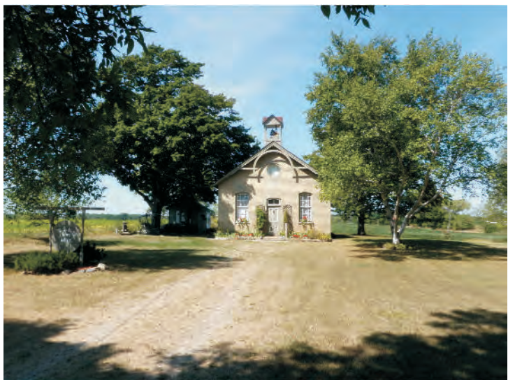
Plate 6 Former Schoolhouse on Blackbush Line, View West
