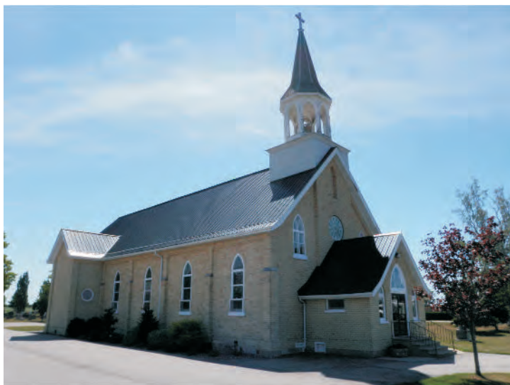
Plate 5 St. Peter's Catholic Church, View Southeast
