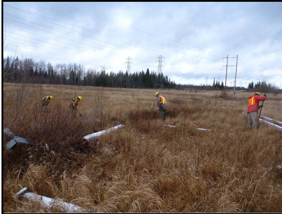
Image 5: View of Crewmembers Test Pitting at 5 m Intervals (Photo Taken on November 16, 2011; Facing Northwest)
