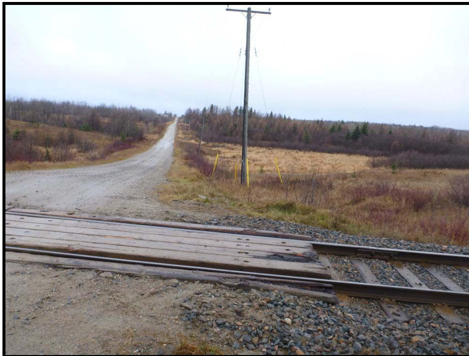
Image 16: Area of No Archaeological Potential – Visibly Disturbed (Photo Taken on November 15, 2011; Facing West)
