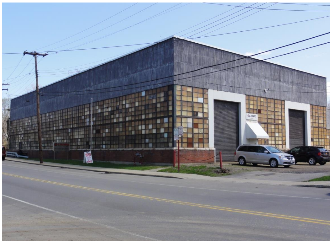
Photograph 6.13. Plant No. 2, S. Howes Inc., facing northeast ( Panamerican 2013 ).
