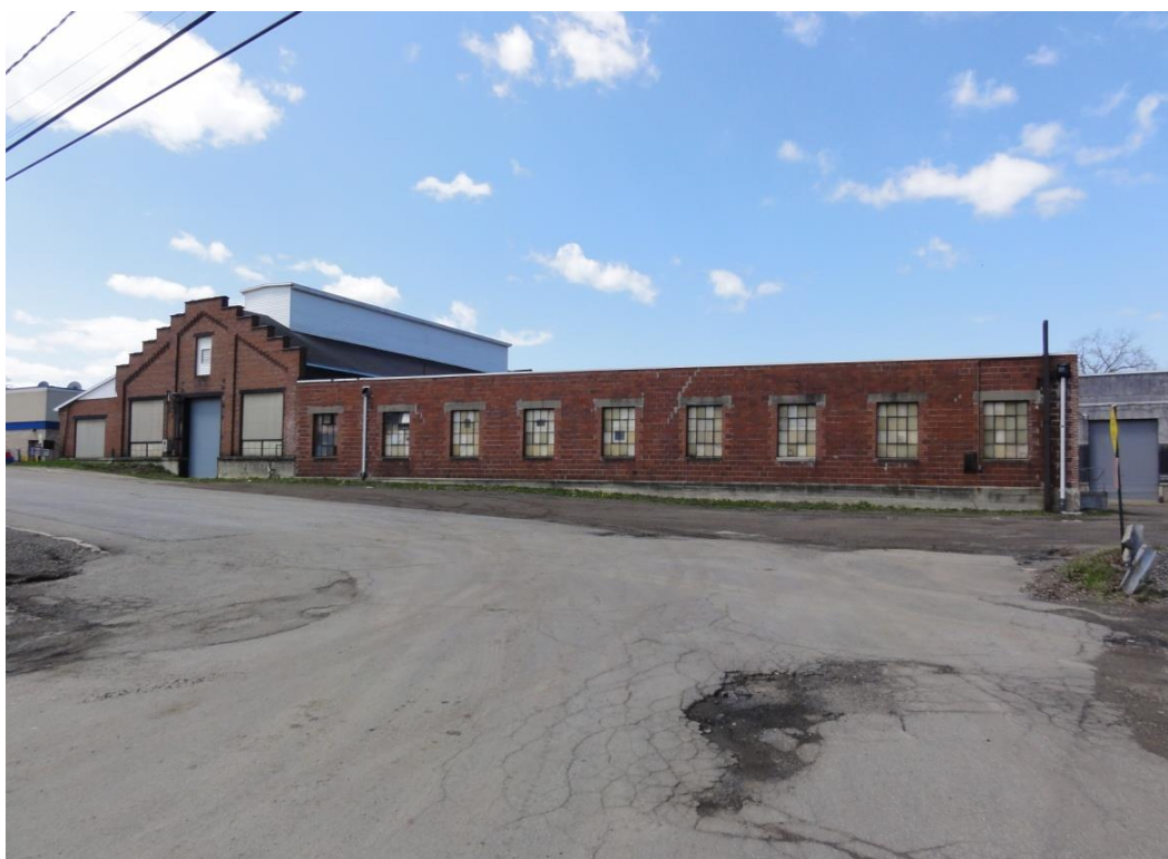
Photograph 6.14. Plant No. 1 and warehouse on North Main Street, Howes Inc., facing southwest ( Panamerican 2013 ).
