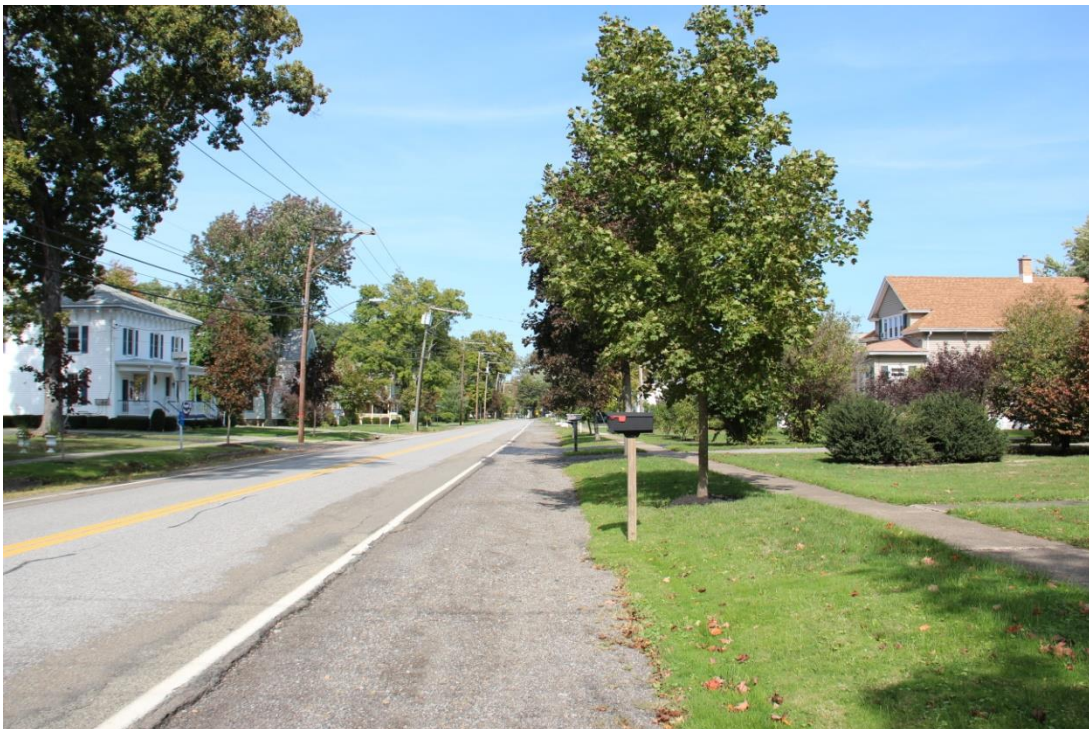
Photograph 6.4. Center Street from 7 Center Street with 9 Center Street at right and 10 Center Street at left, facing north ( Panamerican 2012 ).
