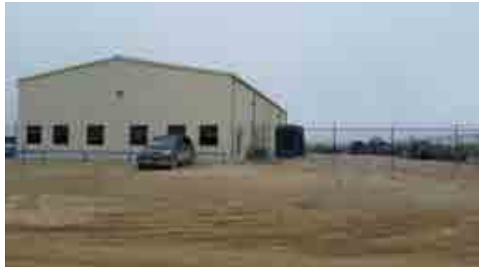
Typical O&M Building and Side Yard
