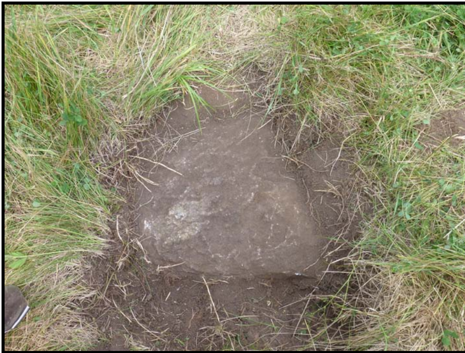
Plate 8: View of Foundation Wall Corner
