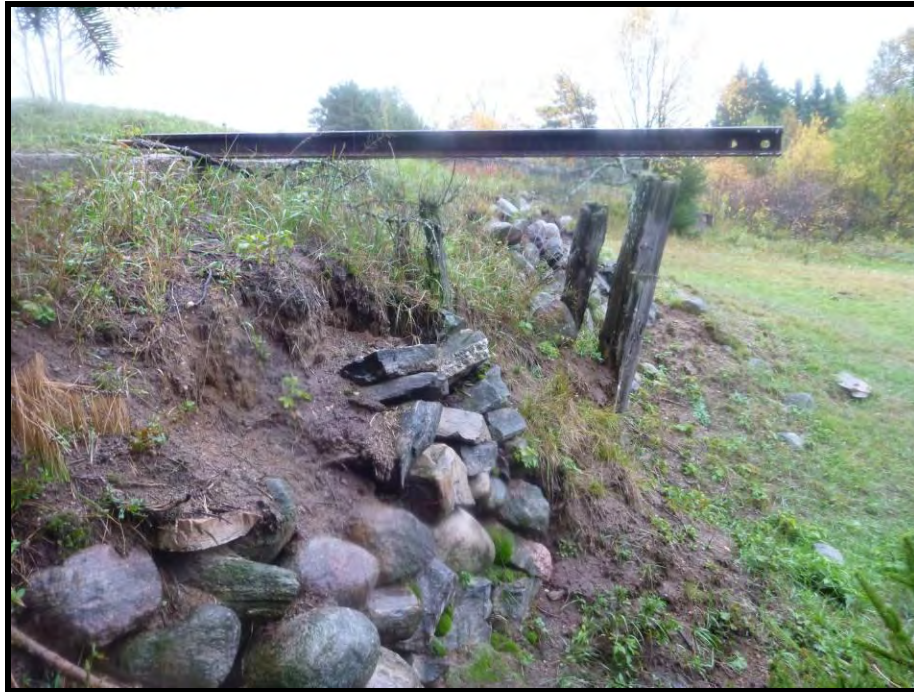
Plate 17: View of Retaining Wall and Track Segment, Facing East
