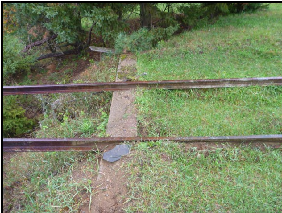
Plate 16: View of Concrete Foundation Supporting Track Segment, Facing West
