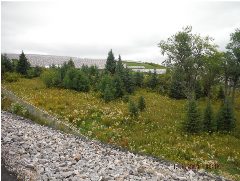
Figure 4 Looking Westward from Substation along Transect C
