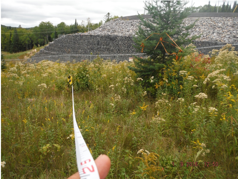
Figure 3 Looking Westward towards Substation along Transect C
