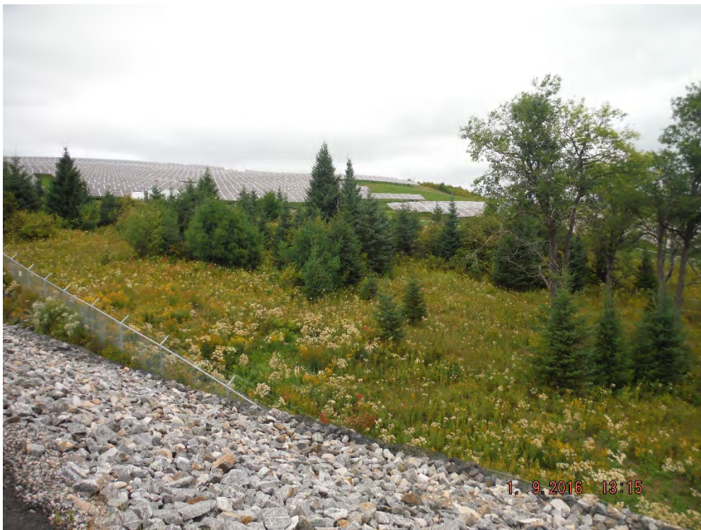
Figure 4 Looking Westward from Substation along Transect C
