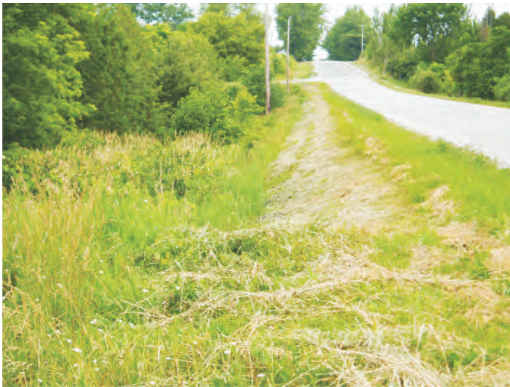
Plate 39 Proposed Transmission Line, West Side Bronson Line, View North
