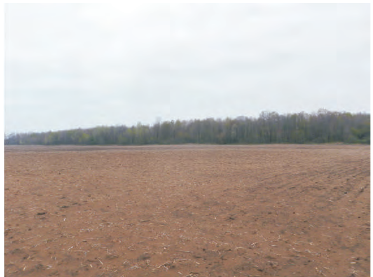
Plate 16 Turbine 25 Pad, View Northwest (May 1 2012)
