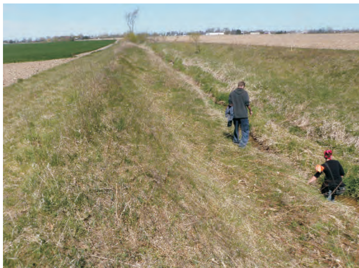
Plate 31 Kading Drain in Access Road Between Turbines 32 and 35, View West Southwest (April 25 2012)
