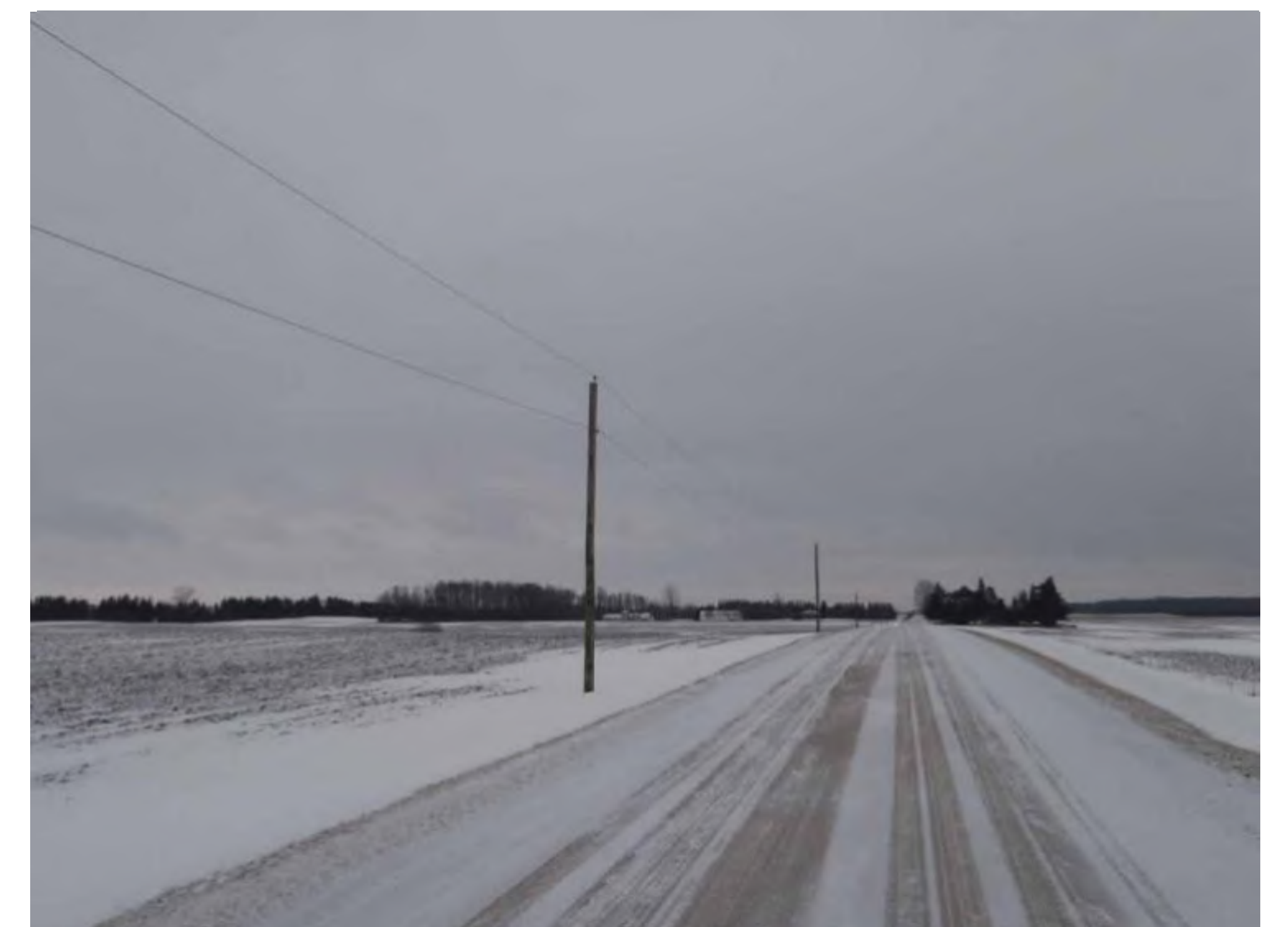
Both photos show existing infrastructure along northern transmission route
